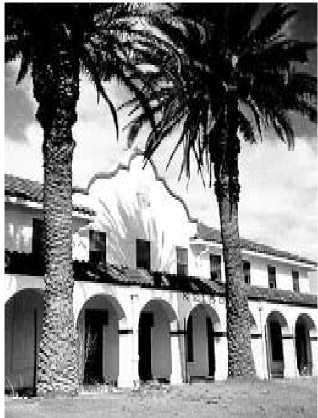
Kelso Depot under restoration. National Park Service photo, 1998.
