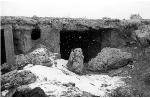
Figure 7. Erosion exposes the thick, dense, mid-Pleistocene pedogenic carbonate at the Valley Wells copper smelter. When the smelter was receiving ore from the Copper World mine, dug out cabins were excavated under the solid carbonates.
